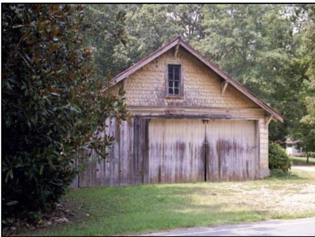
This garage was constructed about 1920 on the Shields-Ethridge farm in Jackson County (Piedmont Region). It has concrete block walls, wooden doors, and an unusual wood shingle design in the gable.
