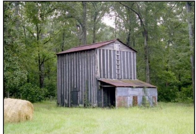
The photograph above shows a 1920s flue-cured tobacco barn in Effingham County with an attached shelter for the exterior furnace. The photograph below is a tobacco barn in Berrien County with wide overhanging sheds (shade skirts) for the stripping process. Both are located in the Central Coastal Plain.
