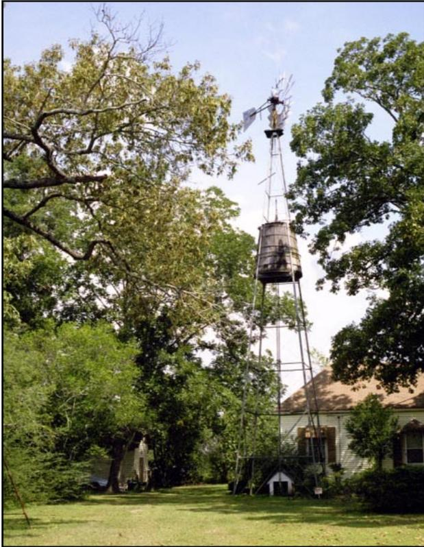
This structure combines a windmill with a water tank within its structure (Sumter County, Upper Coastal Plain). Water was stored in elevated tanks to ensure a gravity flow.
