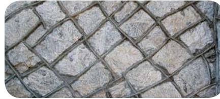
GRANITE WITH BEADED MORTAR JOINTS
