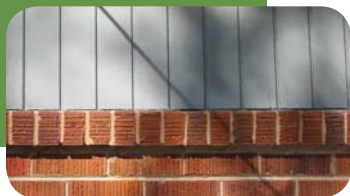
VERTICAL BOARD AND BRICK SKIRTWALL
