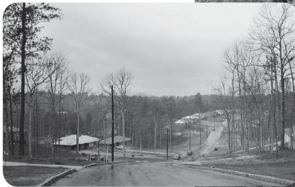
(Above) Construction of the Argonne Forest subdivision in 1955, Fulton County, Georgia. (Source: Georgia State University, Pullen Library, Lane Brothers Photographic Collection). (Right) 1955 Aerial View, North Druid Hills Area Showing Suburban Growth, DeKalb County.
