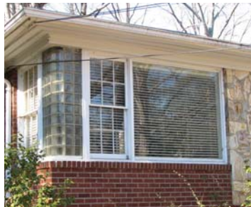
FIXED, SASH AND GLASS BLOCK UNIT
