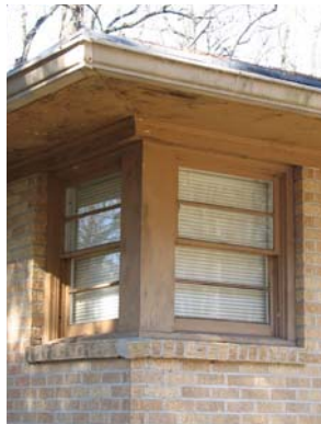
CORNER DOUBLE-HUNG SASH
