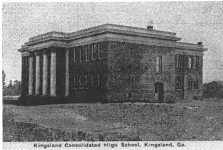
Illustration 16. Two rural consolidated high schools in north (top) and south (lower) Georgia. The photograph of Starr High School is from the Board of Education Reports. The picture of Kingsland Consolidated High School was taken from Camden's Challenge: a history of Camden County, Georgia , p. 113.
