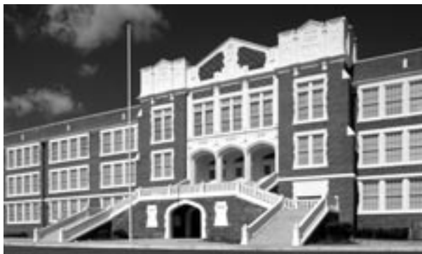
The recently rehabilitated Academy of Richmond County (circa 1925) continues to serve its community as a public high school.
