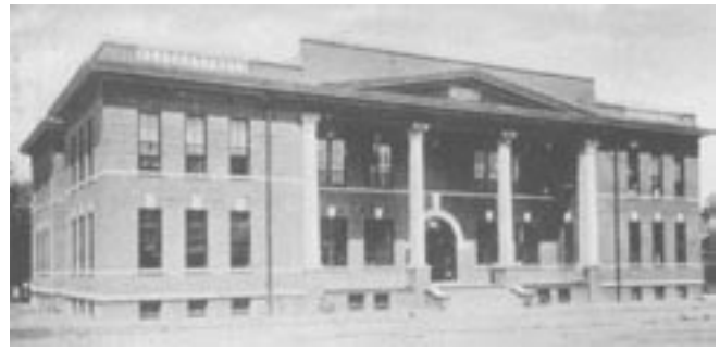
Designed by Columbus architect T.W. Smith, the Valdosta High School was constructed in 1905. The structure functioned as a school until its demolition in the mid-1970s.
