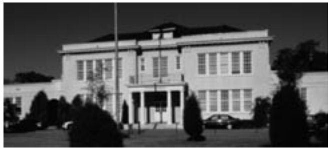
The Wynnton Elementary School in Columbus was built in 1923 around the earlier 1843 Wynnton Academy, a one-room building that now is used as the elementary school's library.
