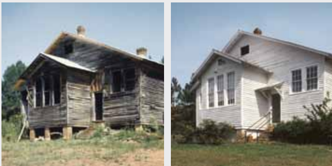
Noble Hill School in Cassville before and after rehabilitation. Courtesy of the Georgia Department of Natural Resources.
