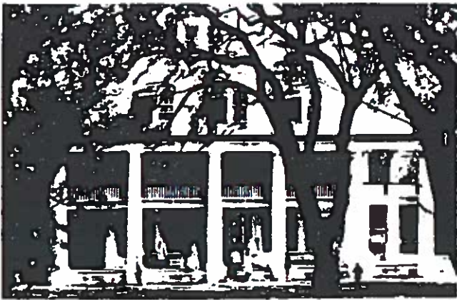
Figure 3. Southern mansions typify climate conscious design. The wide roof overhangs, exterior porches, shade trees, heavy masonry walls (painted white), and living quarters on the second floor (to catch evening breezes and escape the radiant heat from the earth's surface) all are energy saving characteristics which provide reasonably comfortable living spaces without mechanical air conditioning. (Photo: Marcia Astmann Smith)
