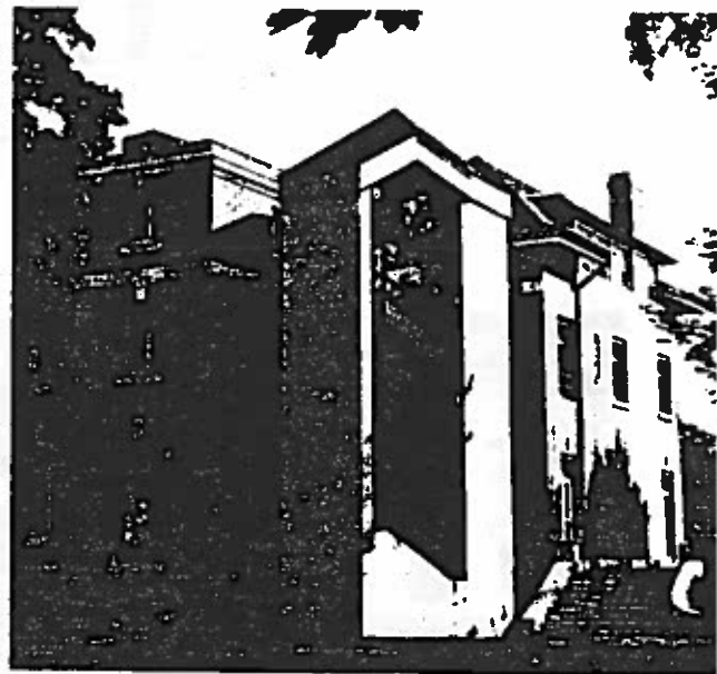
Historic university building with incompatible new stairtower addition. This approach changes the historic character.
