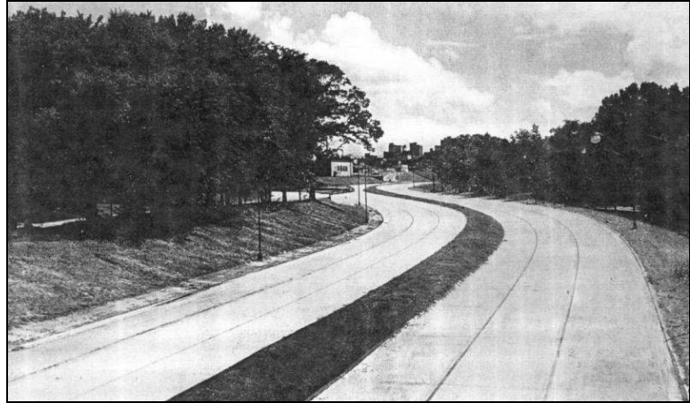
Figure 5. Atlanta Expressway, ca. 1952. The early design standards did not include such features as wide medians, improved shoulders, and lengthy acceleration and deceleration ramps that would be required of post-1956 interstate highways. Nonetheless, the pre-1956 roads were incorporated into the interstate highway system with plans to upgrade them at a later date. Source: Biennial Report (1952).
