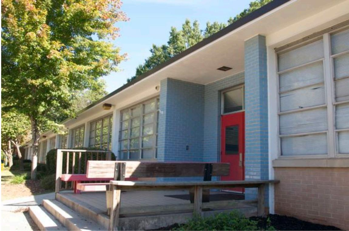
Figure 55: Use of blue glazed brick on secondary entrance at Montgomery Elementary
