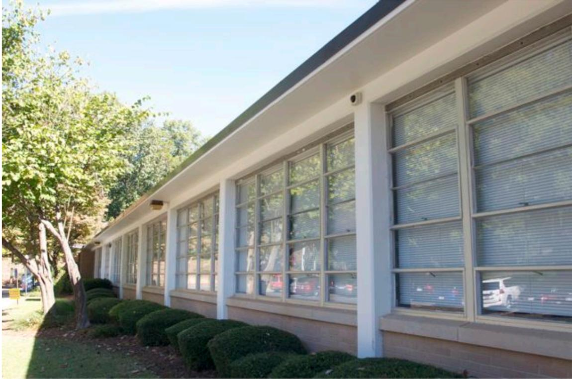
Figure 51: Beige brick and awning/hopper windows at Montgomery Elementary
