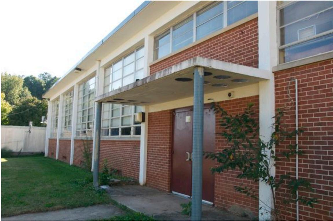
Figure 33: Flat overhang with circular cut-outs at Gresham Park Elementary
