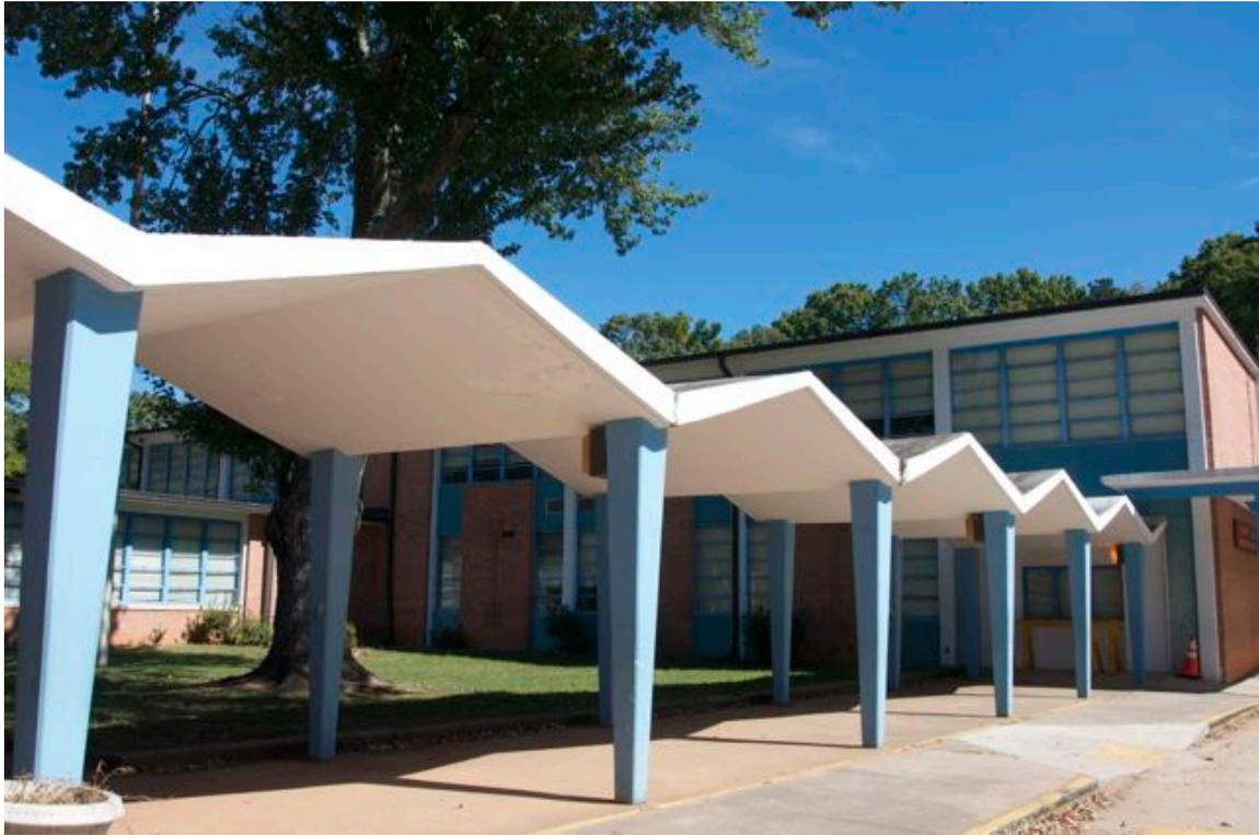
Figure 46: Zigzag canopy at Columbia Elementary
