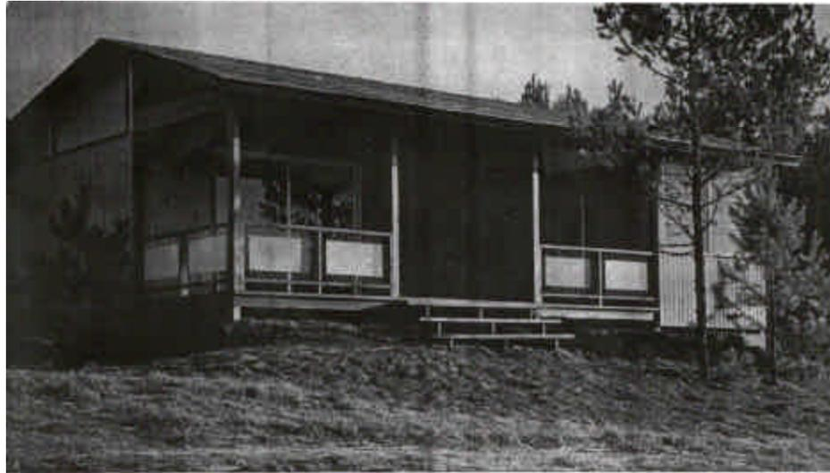
Prefabbed vacation house—designed to sell for \$3,000 to \$5,000 without land—is erected on steel/wood posts in precast concrete footings.
