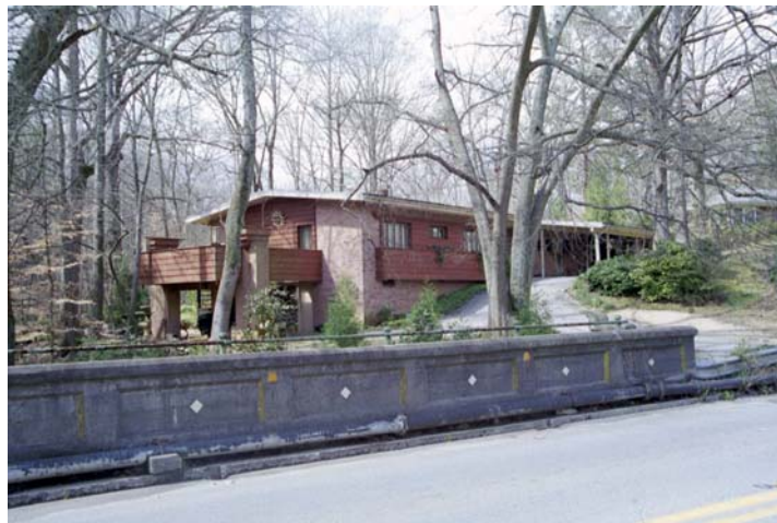
Figure 70: Near Howell Mill Road, Atlanta, Georgia
