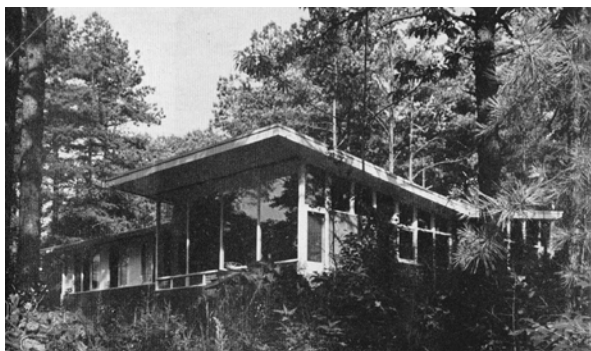
Figure 35: Wilkinson Residence, West Paces Road (razed) S&W 1919-1948 p.102-103. Designed as passive solar home.
