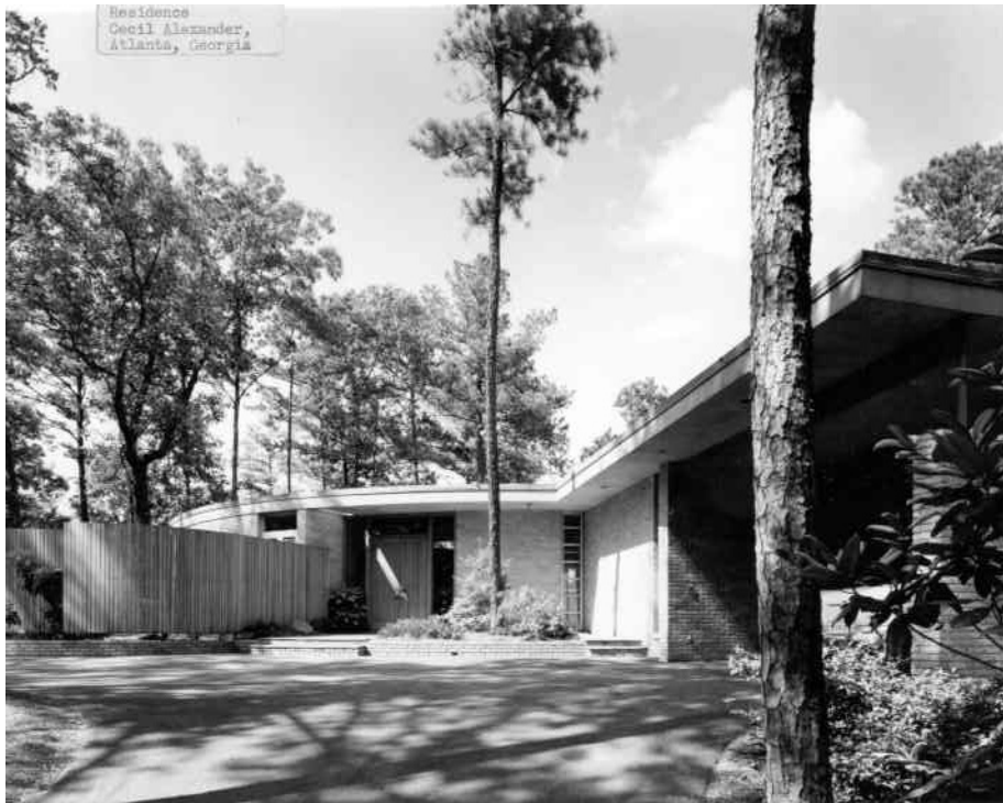
Figure 19: Alexander Residence, 2322 Mt. Paran Road. Published The South Builds , p.38 This house has an unusual round plan. Firm: Harrison & Abramovitz, Toombs Amisano & Wells
