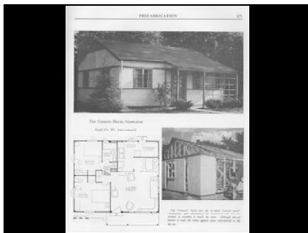
While this “cemento” house was built with prefabricated cement-and-asbestos panels.
