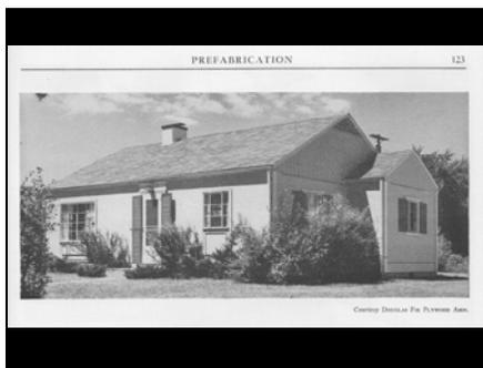
In some parts of the country, American Small Houses were built using experimental construction materials and techniques. This house was built using plywood for the exterior sheathing ...
