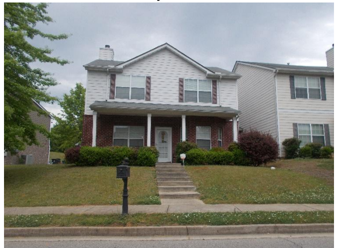
Single-family homes northeast of the Subject site
