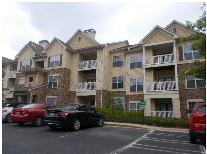
Stillwood Farms Apartments (included) south of the Subject site
