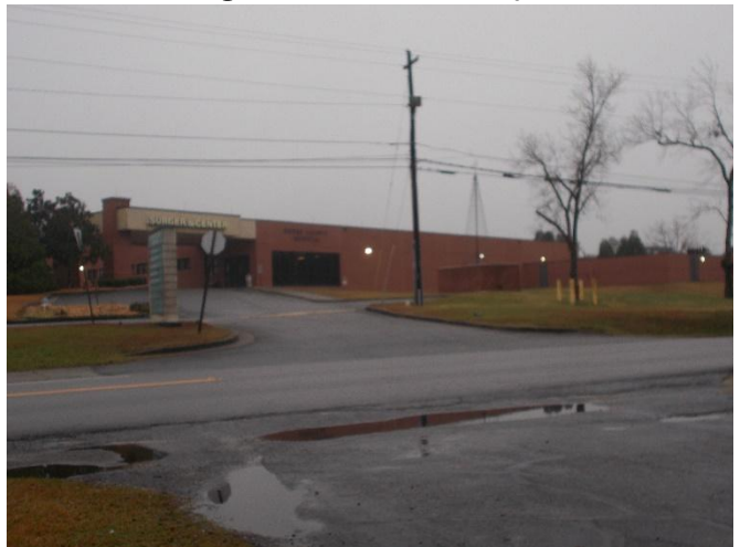
Hospital west of Subject site
