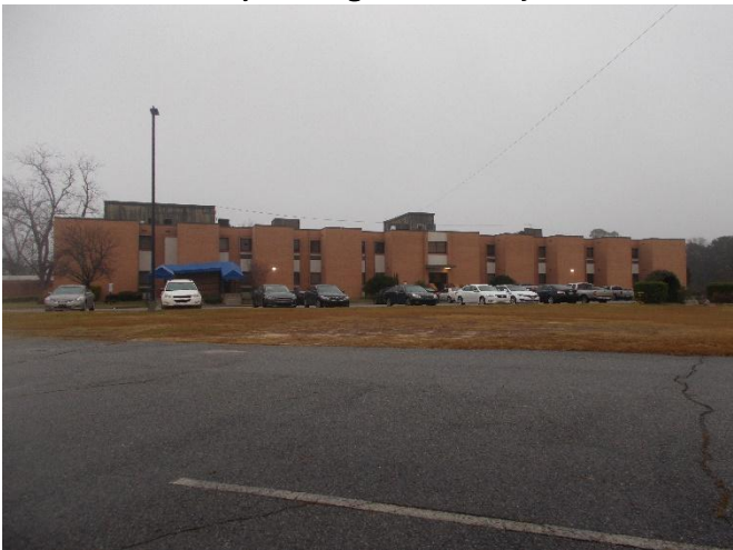
Hospital west of Subject site
