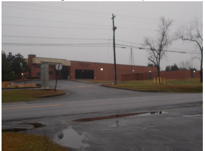
Hospital west of Subject site
