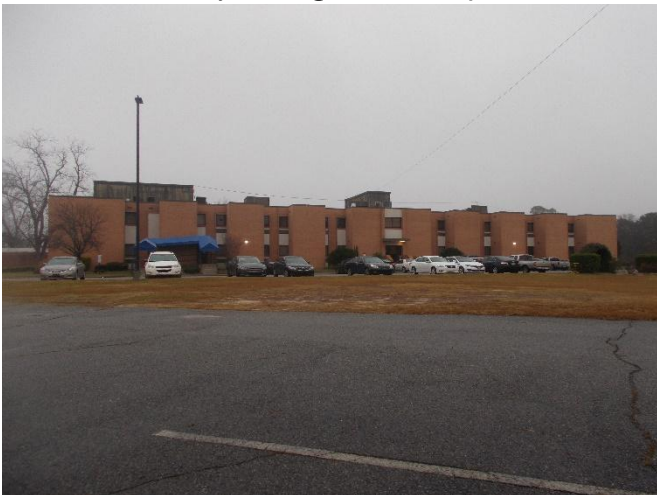
Hospital west of Subject site
