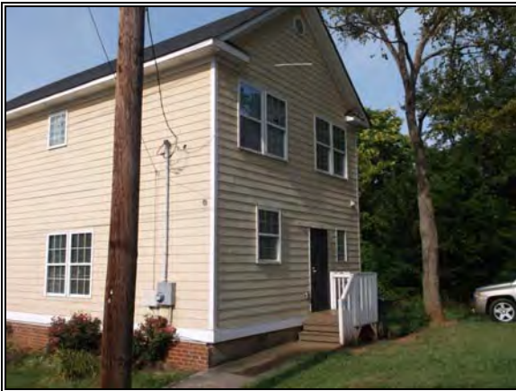
Northern Side Of Single-Family Residence
