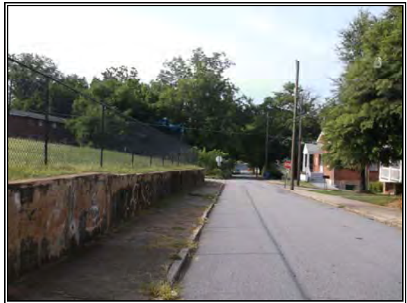
Southerly View Along Walnut Street, Subject On Right
