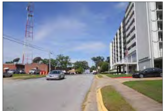
Looking West from Entrance
