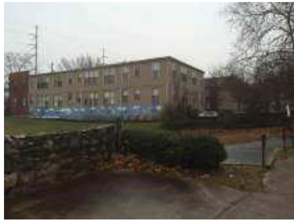
Bedford Pines V (HUD Section 8 community) bordering the site to the south
