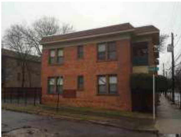
Bedford Pines I bordering the site to the west
