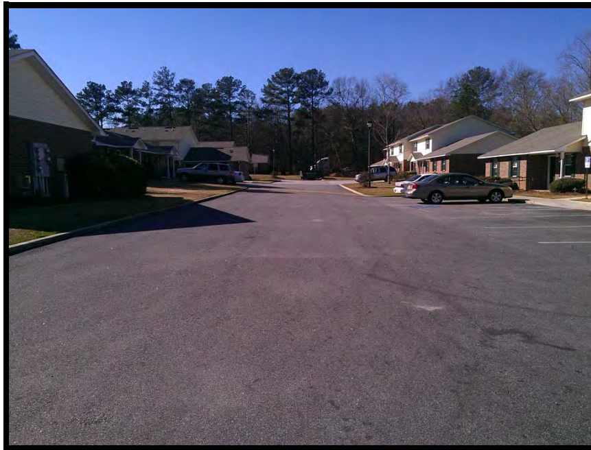
Typical Site Streetscape
