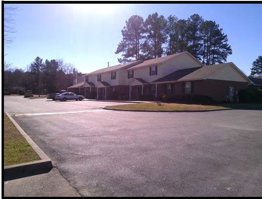
View of site from the northeast
