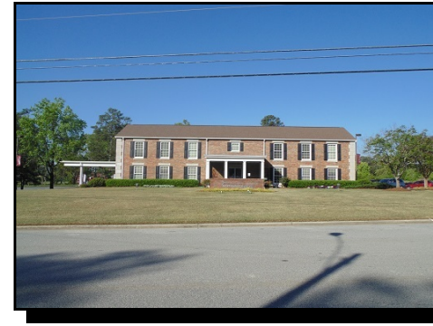
(10) NW Georgia Credit Union, .1 mile from site.
