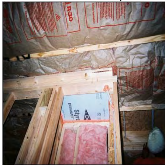
CORRECT: Well-sealed Chase (Prior to Duct Installation)
