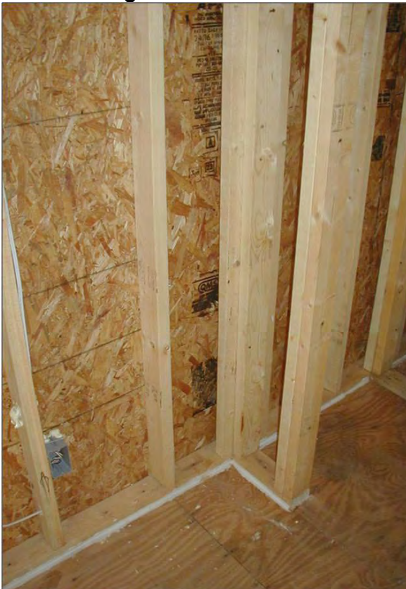
Caulking Around Bottom Plate
