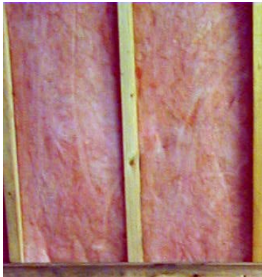
CORRECT: Batt in Wood-framed Cavity
