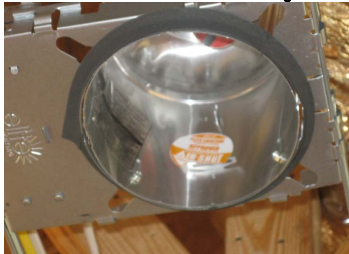
CORRECT: IC-Rated and Air-Tight
