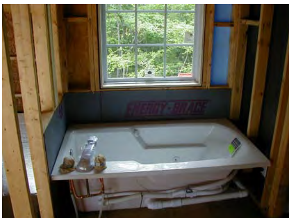
CORRECT: Air Barrier and Insulation Behind Tub
