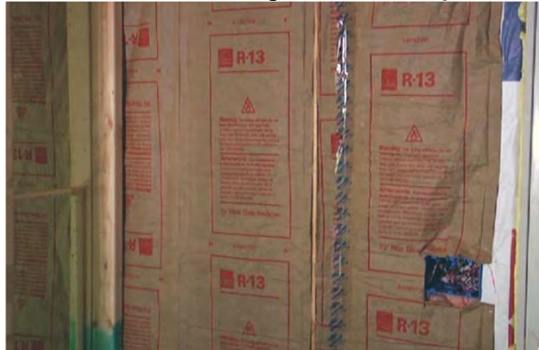
CORRECT: Full Coverage and No Compression
