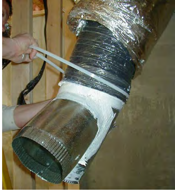
CORRECT: Mastic-sealed Joints
