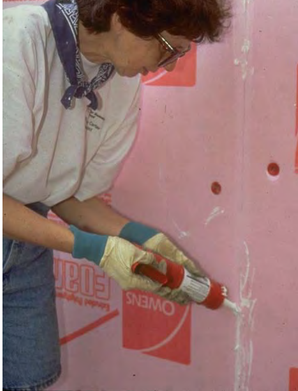
CORRECT: Sealing Exterior Sheathing
