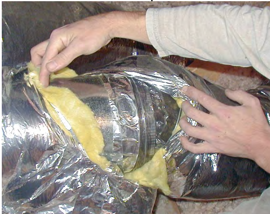
INCORRECT: UL-181 Tape without Mastic
