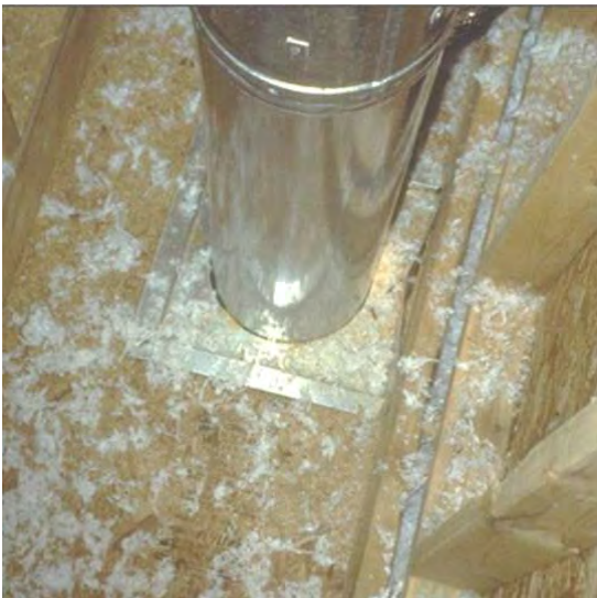
CORRECT: Well-capped Chase
