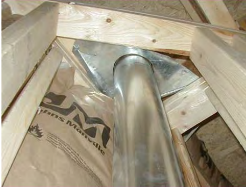
CORRECT: Well-capped Chase
