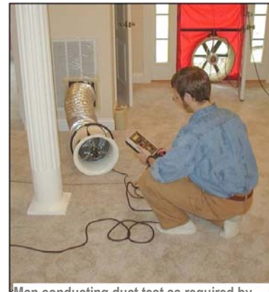
Man conducting duct test as required by Georgia energy code.
