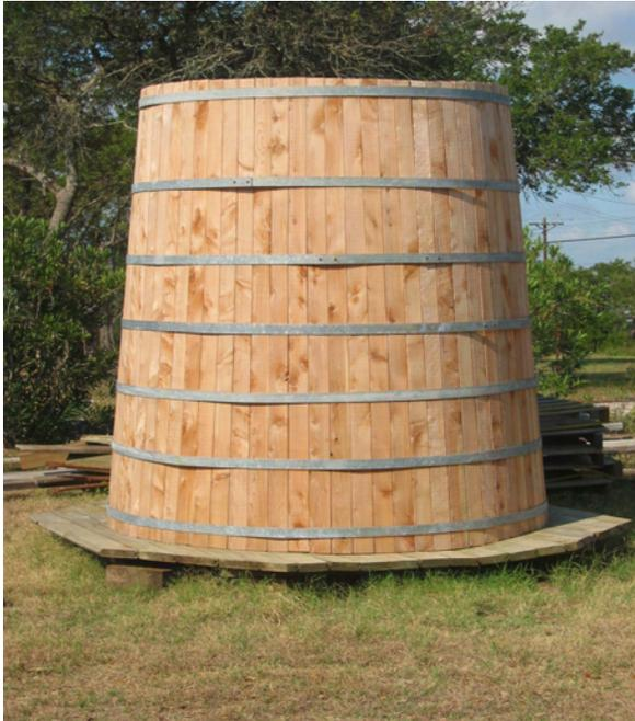
Figure 4.15 Wooden aboveground tank
