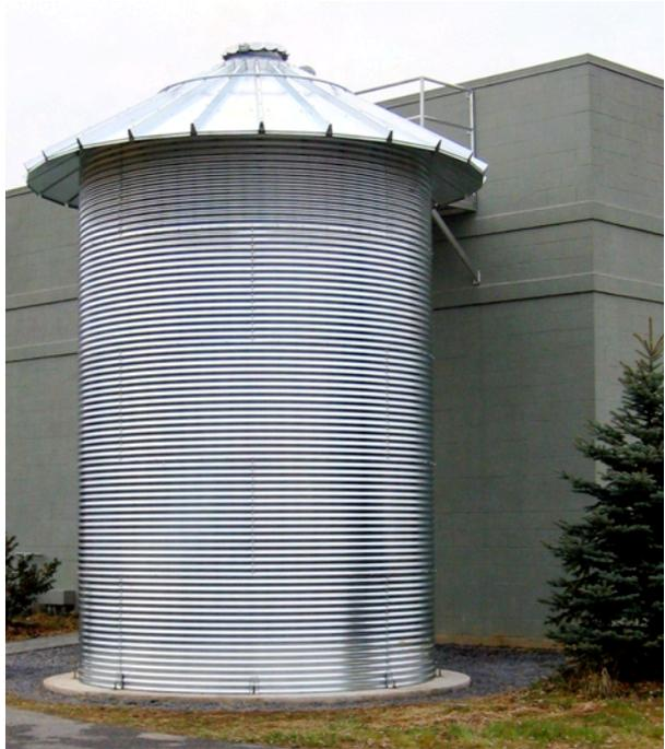
**Figure 4-14 Corrugated steel tank**
