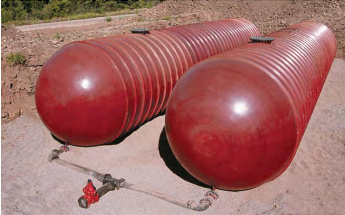
**Figure 4.12 Below ground fiberglass tanks**
