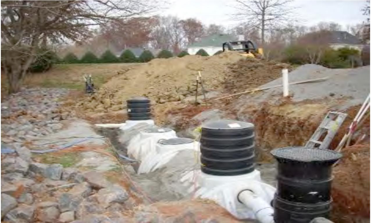
**Figure 4.13 Below ground polypropylene tanks**
