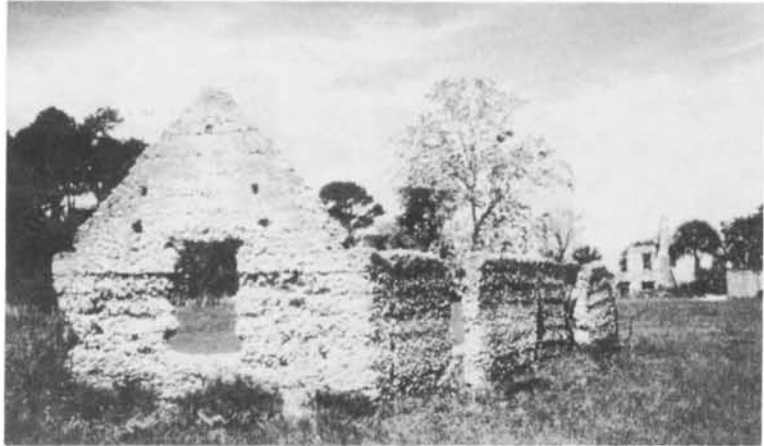
Chocolate Plantation on Sapelo Island in McIntosh County is believed to have been built sometime between 1812 and 1820. The site consists of over fifteen tabby structures, including the main house, individual slave cabins (above), storage buildings, an infirmary, and stables.
