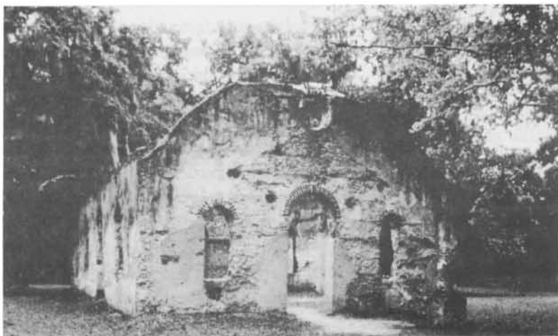
The Saint Helena Chapel of Ease (circa 1740) features tabby walls with brick columns and brick arches over the window openings.
