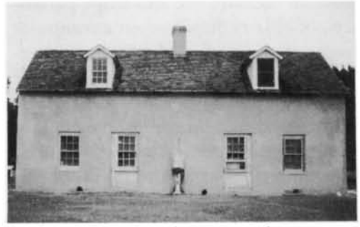
The Tabby House, front and rear elevations, nearing completion. The completed walls are drying to a uniform, warm, light brown color (Munsell Colour 10YR 8/1), closely matching the original color. Photographs by Melanie Taves.
