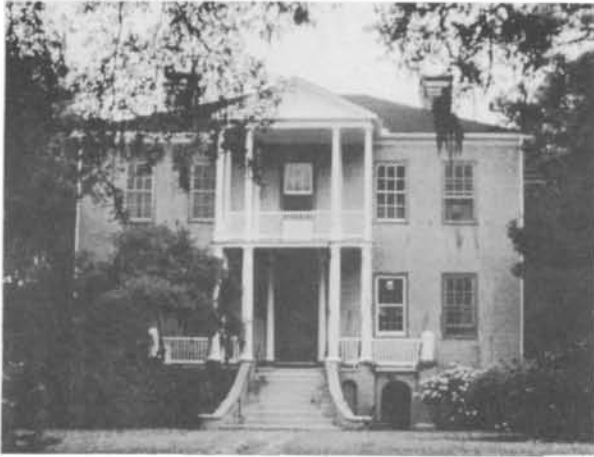
Dating from 1787, Tabby Manse in Beaufort, South Carolina, has two-story tabby walls on a raised tabby foundation.
