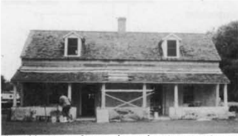
The Tabby House, front and rear elevations, nearing completion. The completed walls are drying to a uniform, warm, light brown color (Munsell Colour 10YR 8/1), closely matching the original color. Photographs by Melanie Taves.
