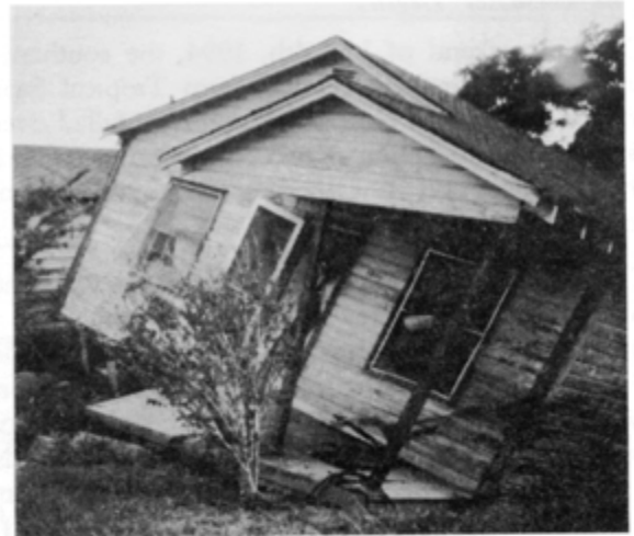
Hundreds of historic buildings like this residence suffered damage from rain, flood, sinkholes, mud and mildew.
