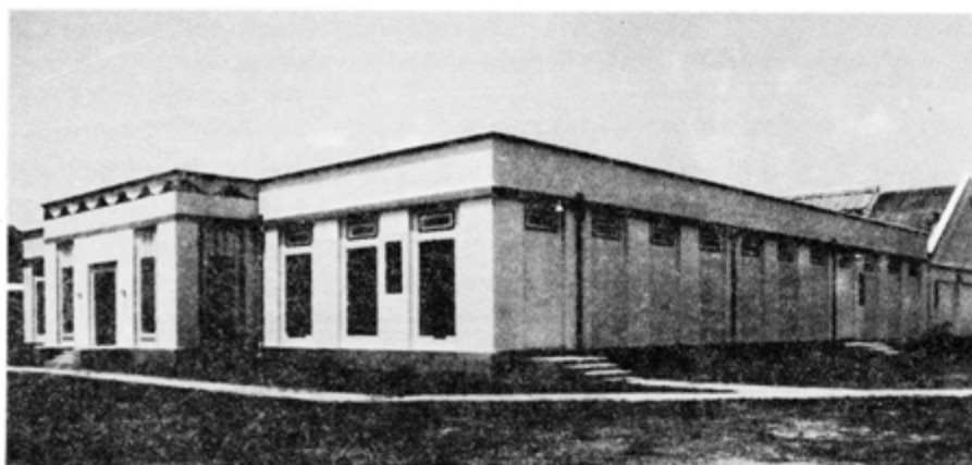
The historic Macon Water Works could be redeveloped as a community park.
