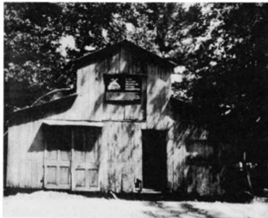
Fielder's Grist Mill was damaged by flood waters surging through its foundation and machinery. Now the mill is operating again at full capacity.
