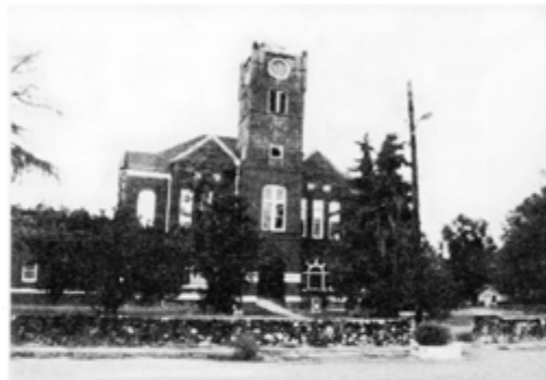
This is how the Baker County Courthouse looked after the flood waters receded.
