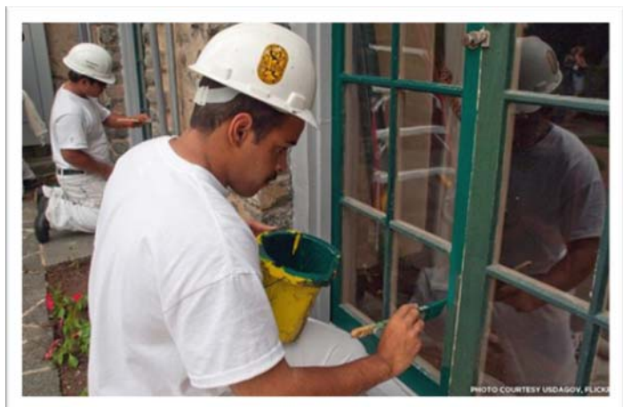
Workers Restoring Historic Windows
