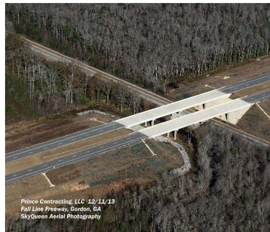
Figure 11 – The Fall Line Freeway has improved diverted thru traffic away from residential areas, but vehicles still travel quickly through many town centers, including on the Fall Line Freeway through Ivey.
