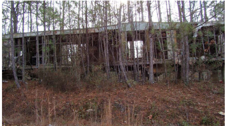
Figure 9 – A dilapidated house in Ivey, shown above.
