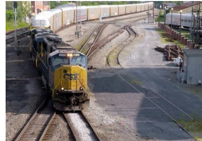
Multiple railways are located adjacent to Dalton's downtown which spurred the need to establish a quiet zone as a method to continue marketing the downtown as a destination for urban and loft dwelling redevelopment
