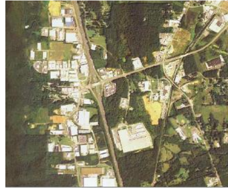
Interchange includes a mix of warehouse, industrial and retail uses in buildings with large, one-story footprints. The area is designed to accommodate automobile traffic, but provides few options for walking and biking
