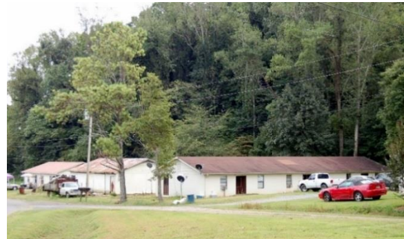
Multi-family residential housing on Mount Olivet Drive
