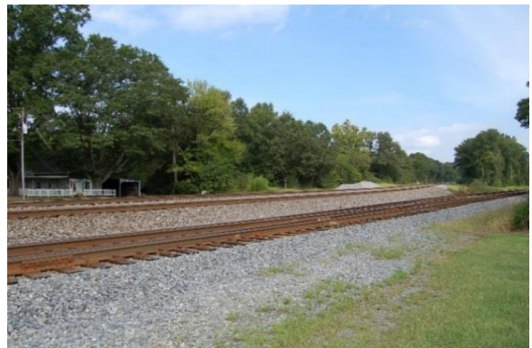
Norfolk Southern rail lines going north out of Cohutta
