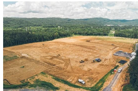
Construction site of Hanwa Q Cells, A global manufacturer of solar panels, in Whitfield County's Carbondale industrial park. This company plans to create approximately 500 new jobs.
