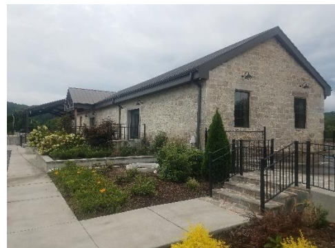
The adaptive renovation of the City's historic train depot has become a tremendous success story. Transformed from near ruins, the depot is now a premier event venue for both city residents as well as the general public.
