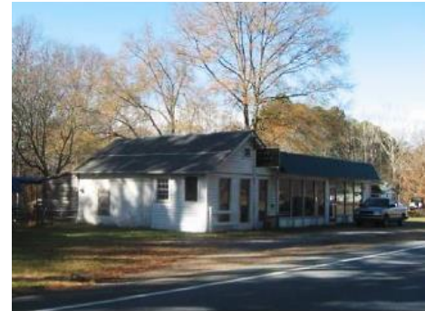
Businesses, such as the one above in north Tunnel Hill on U.S. 41, are an example of the Transition Corridor character area
