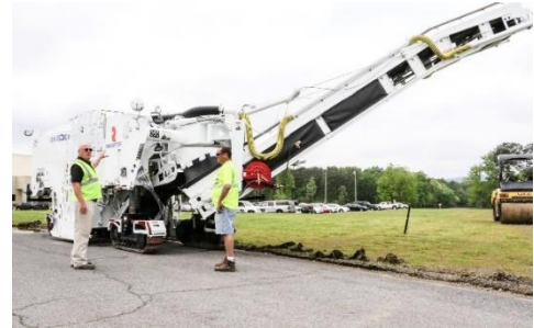
Whitfield County Public Works Director, showcasing the county's new milling machine
