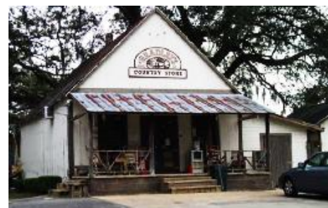
Site design that place parking in the rear or side of buildings help preserve rural character, while also providing retail and other services for surrounding communities
