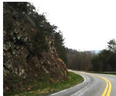
Dug Gap Road winds through the ridge west of Dalton
