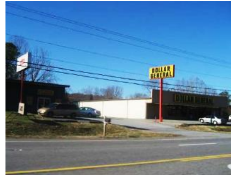
Commercial Development along SR 71/Cleveland Highway in Varnel
