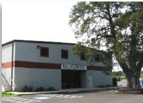
Figure 79: Varnell's Gymnasium provides recreation for area residents
