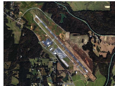
Aerial Image of Dalton Municipal Airport
