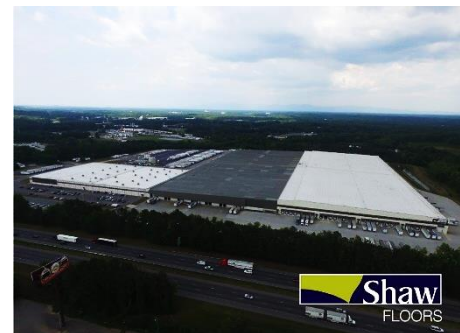
Example of modern industrial property near I-75
