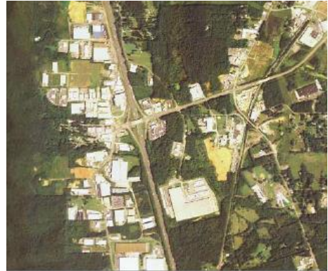
Interchange includes a mix of warehouse, industrial and retail uses in buildings with large, one-story footprints. The area is designed to accommodate automobile traffic, but provides few options for walking and biking
