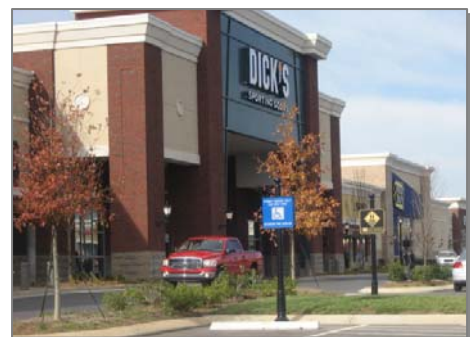
Regional Activity Center example of appropriate scale shown from The Avenue of Murfreesboro in Murfreesboro, Tennessee
