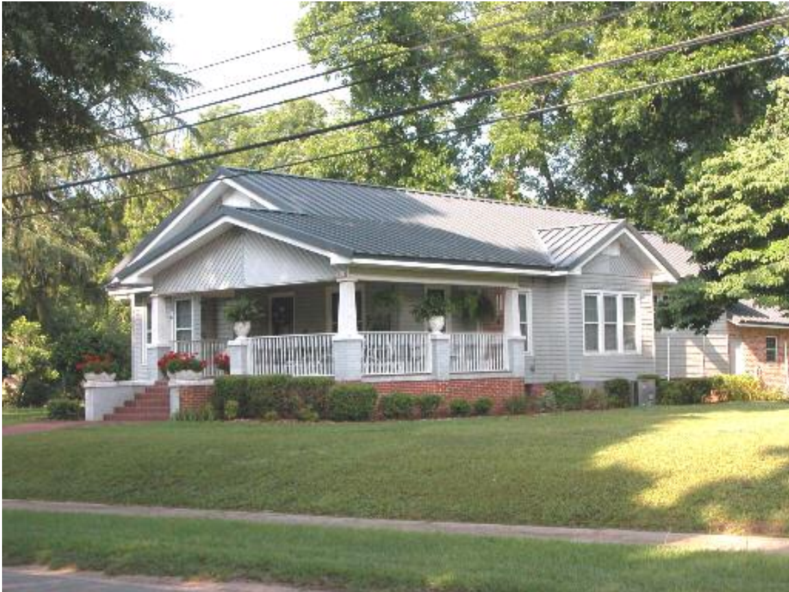
This home, owned by Meridith and Debbie Walker at the time of this report, has undergone extensive renovation with the addition of vinyl siding and a metal roof.
