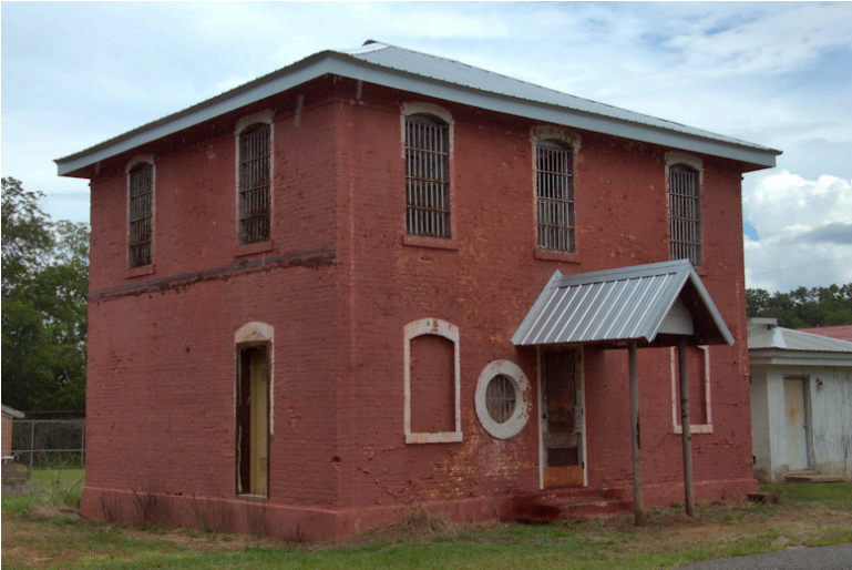
Webster County Jail c. 1910 placed on the National Register of Historic Places in 2000. Photograph Courtesy of Brian Brown, https://vanishingsouthgeorgia.files.wordpress.com
