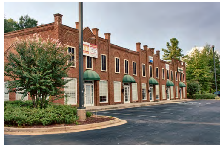
North Point Business Center
