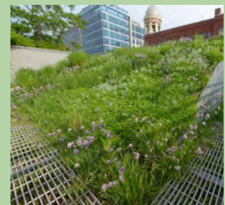
T2-T6: Green roof
