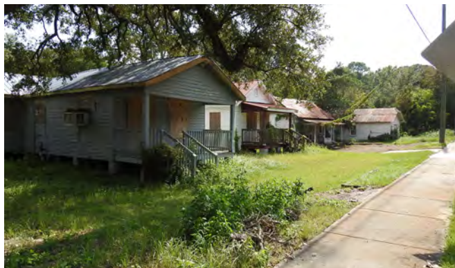
These boarded up and derelict houses are illustrative of many areas of Thomasville. More should be done to limit and stop the increase in these types of properties.
