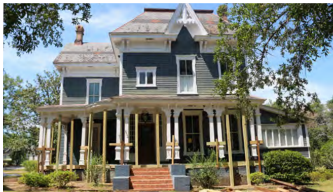
Historic Home Undergoing Restoration
