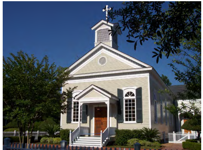
Even small civic buildings can have a dominant presence when properly sited.
