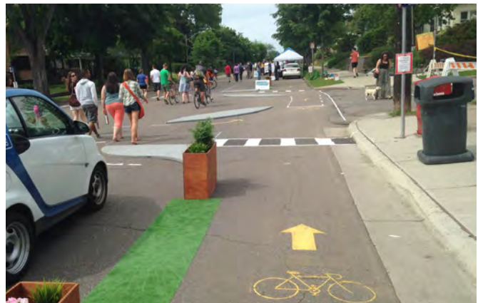
Tactical installations can increase access for pedestrians through bike lanes, landscaping, and parallel parking. These narrow the street and reduce speeding, making the right-of-way safer for pedestrians.
