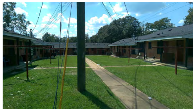
Rear yards also create public spaces which reduces private space. At the same time utility poles and wires detract from the cohesiveness of the development.
