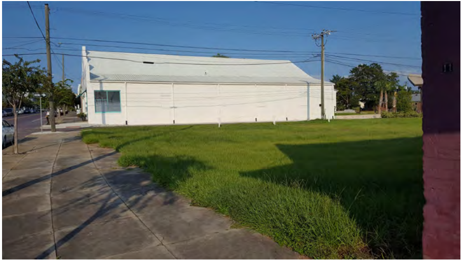
Temporary Interventions: Existing Conditions
