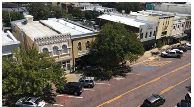
Angled On-Street Parking on Broad Street
