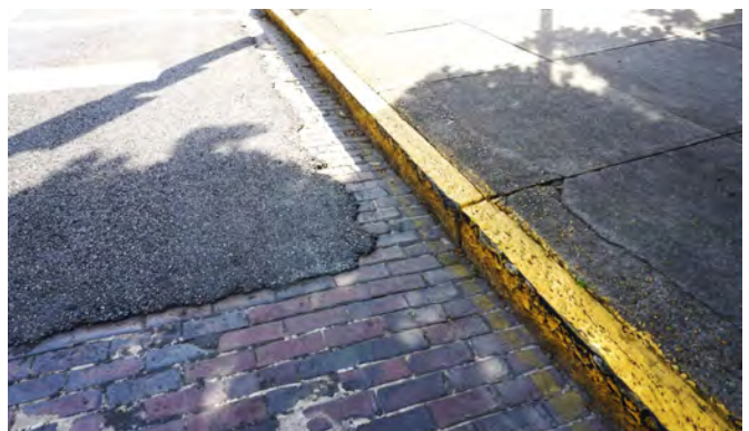
Old meets new - Bricks with granite curbs
