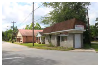
Vacant commercial building
