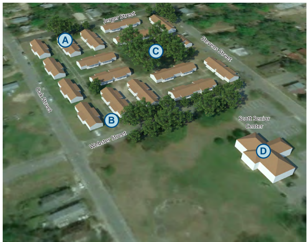
Faircloth Homes: Existing Conditions Aerial
