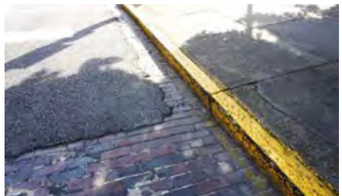
Old meets new - Bricks with granite curbs
