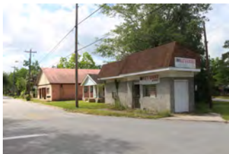
Vacant commercial building
