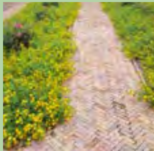
T3-T4: Concrete Paver block
