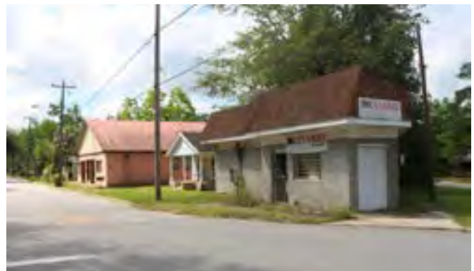
Vacant commercial properties in neighborhood centers
