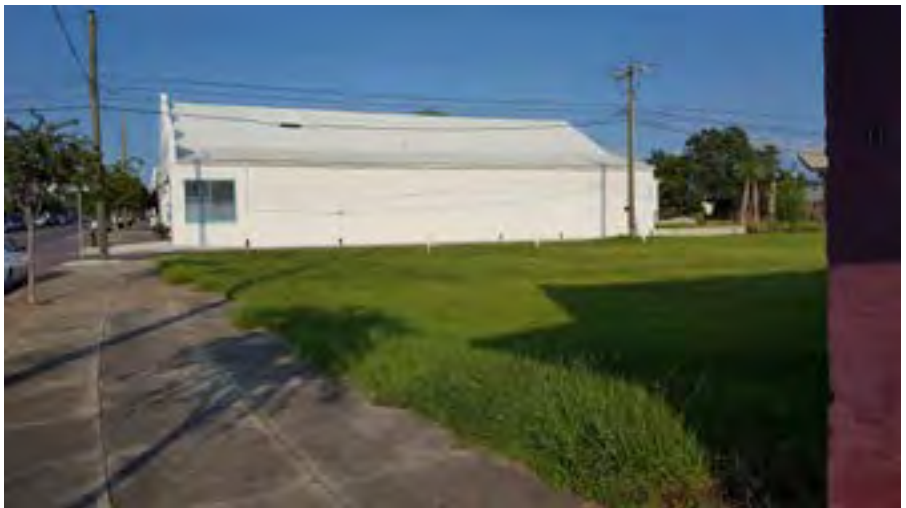
Temporary Interventions: Existing Conditions
