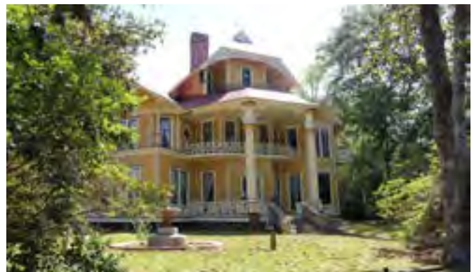
The historic Lapham-Patterson House has porches and large overhangs responding to the local climate.
