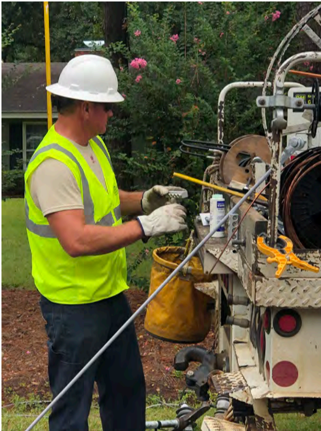
Broadband Service Installation
