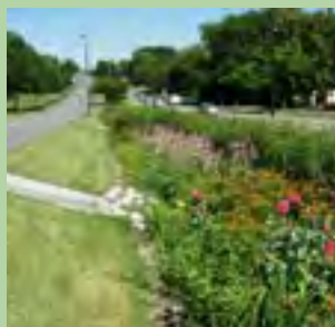
T2-T3: Bioretention swale
