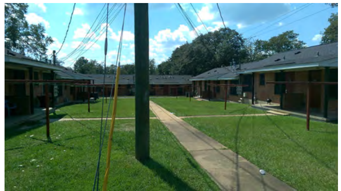
Rear yards also create public spaces which reduces private space. At the same time utility poles and wires detract from the cohesiveness of the development.
