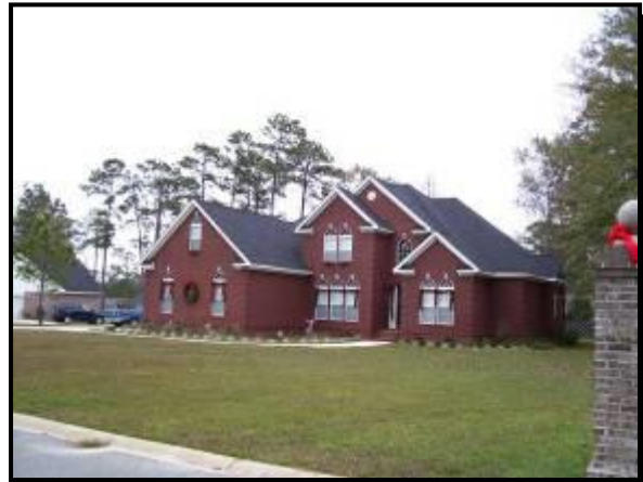
Housing Construction in Thomas County
