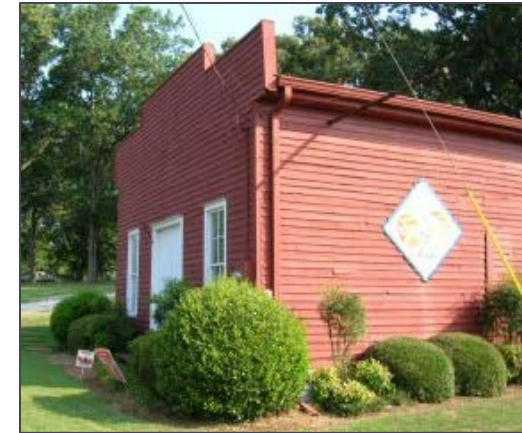
Talmo's General Store is shown on the right and an example of retail design compatible with the small town character shown below.
