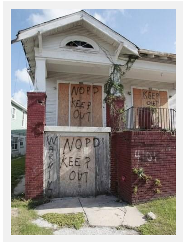
Neglected maintenance can lead to neighborhood blight
