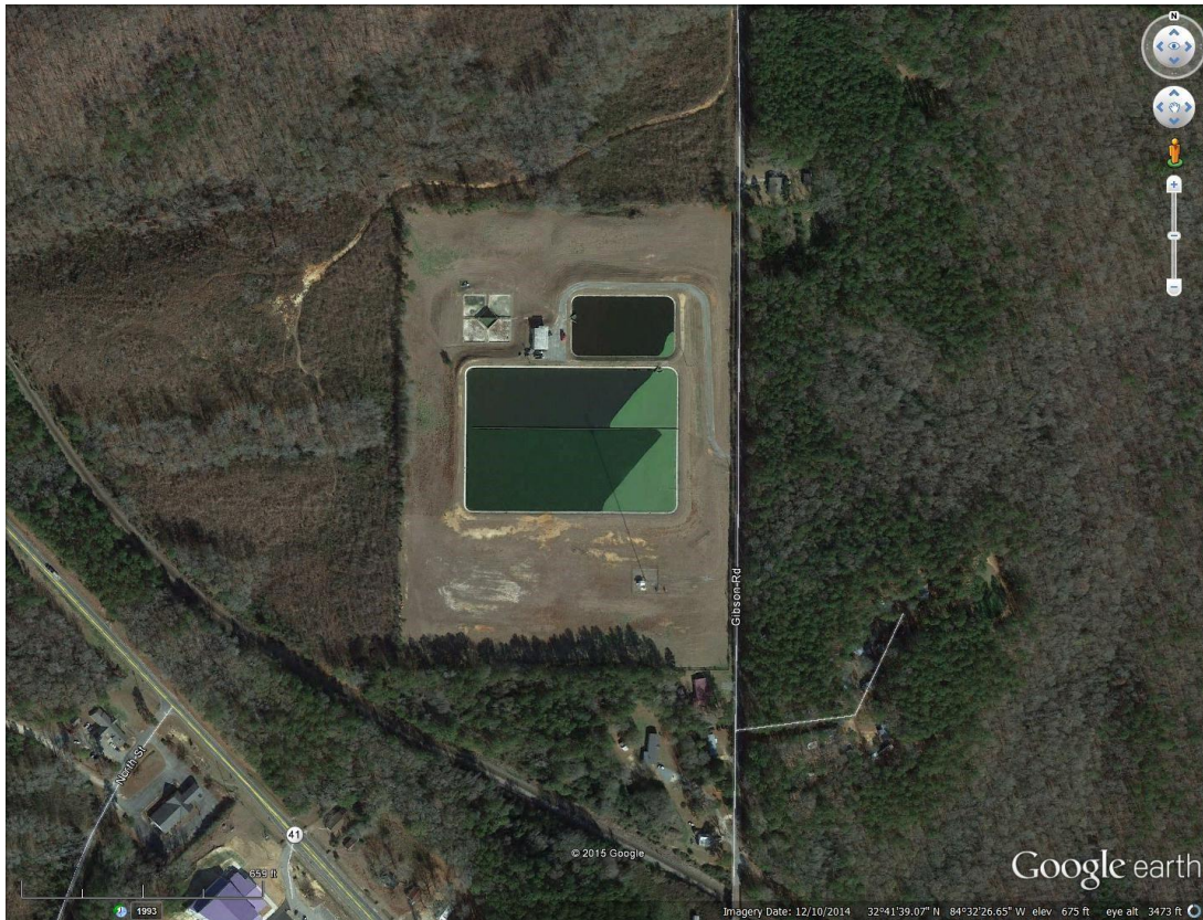
Aerial View of Talbotton's Sewage Treatment Facility on Gorman Road.
