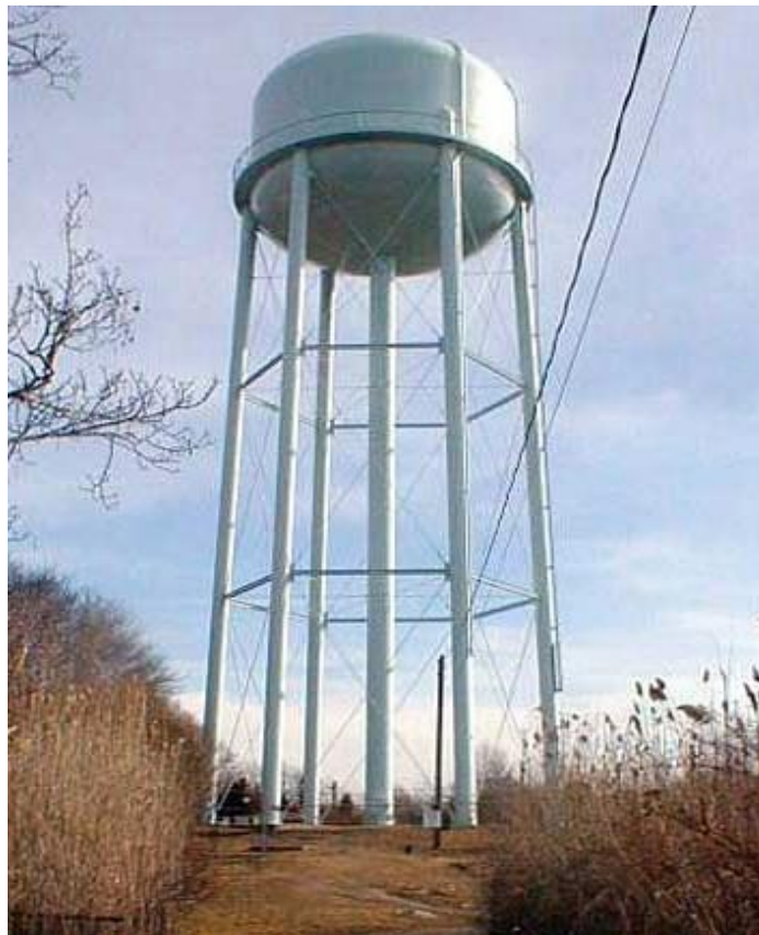
Example of a water tower
