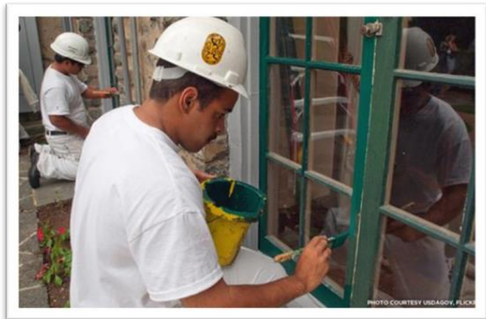
Workers Restoring Historic Windows
