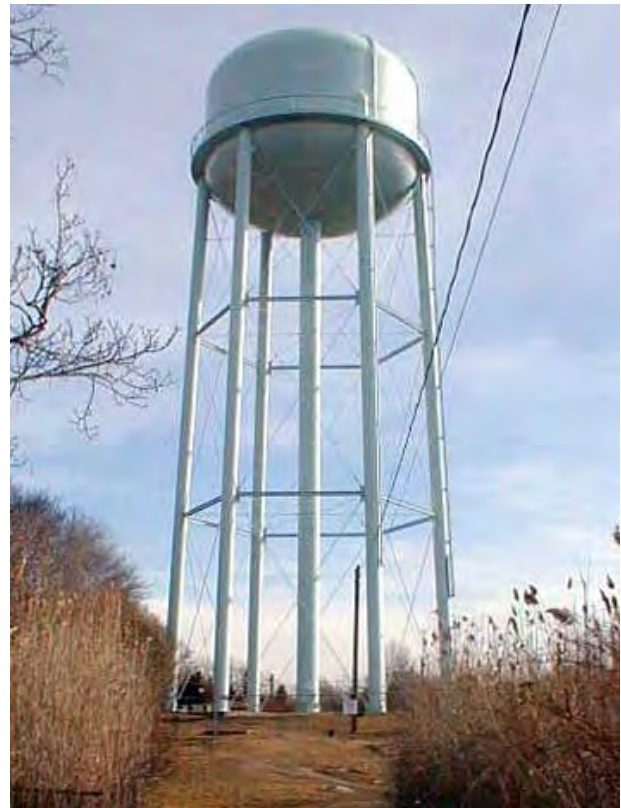
Example of a water tower
