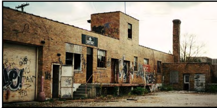
Example of a Brownfield
