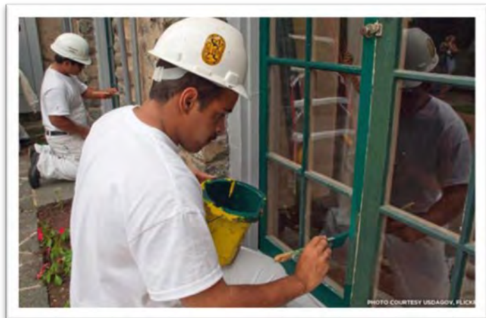
Workers Restoring Historic Windows
