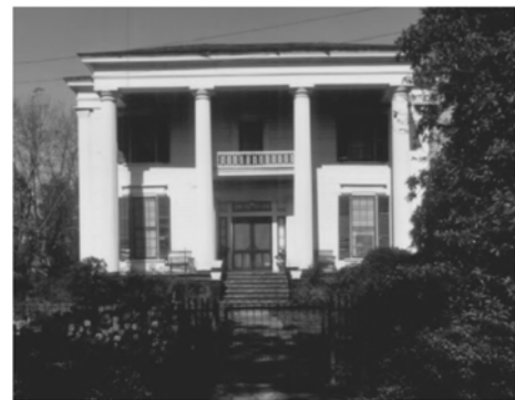
Liberty Hall National Register Listed Property
