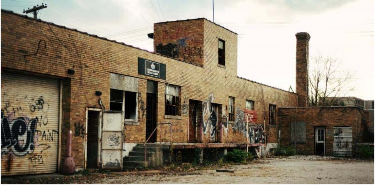
Example of a Brownfield
