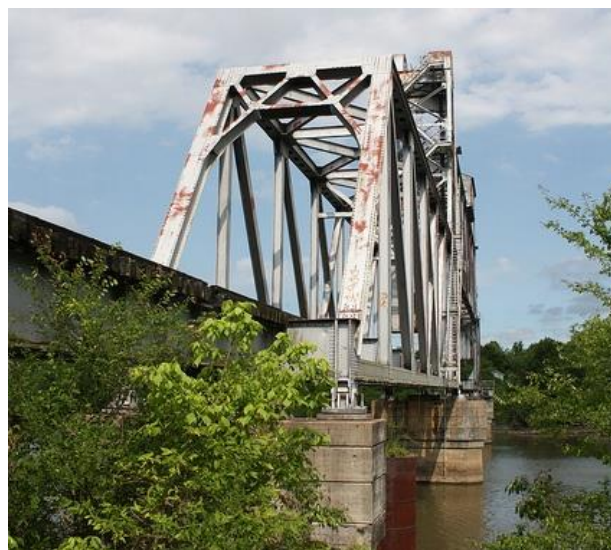
Omaha Railroad Bridge
