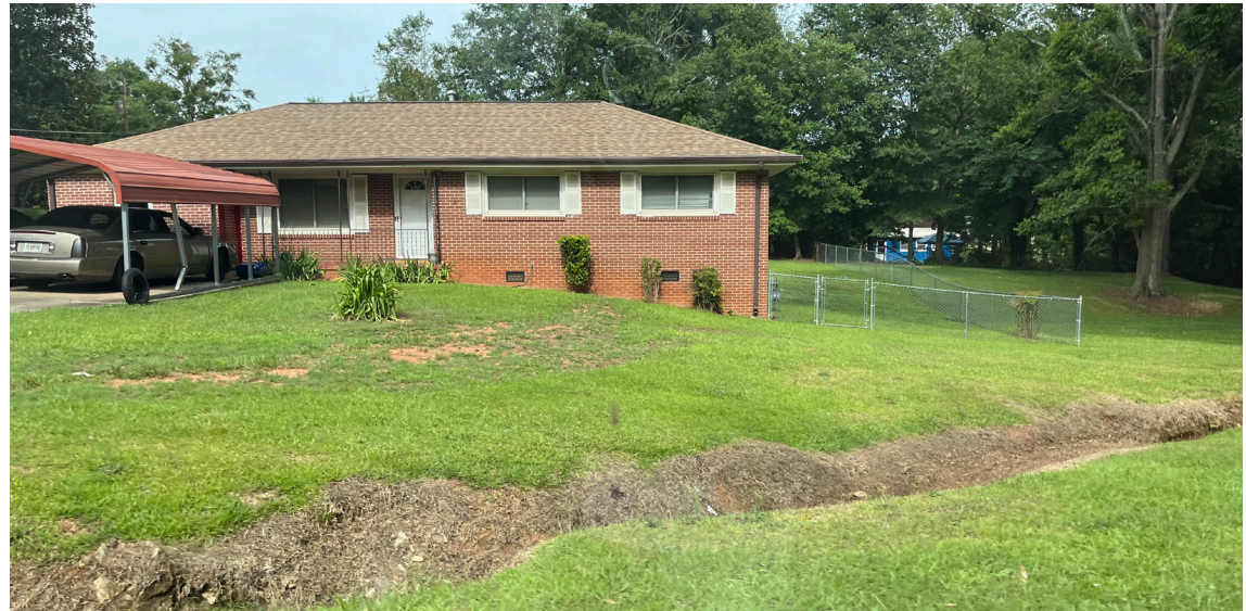
An example of housing in Spalding County that has a drainage ditch in the front yard.
