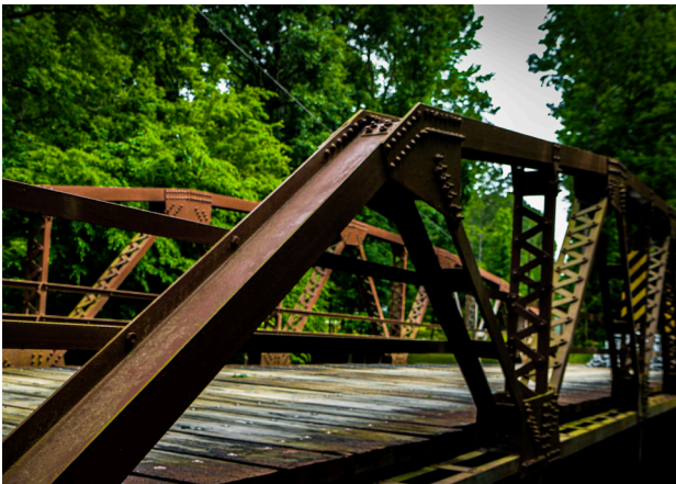
Jenkinsburg Bridge, a historic truss bridge on Jenkinsburg Road, over the Towaliga River.
