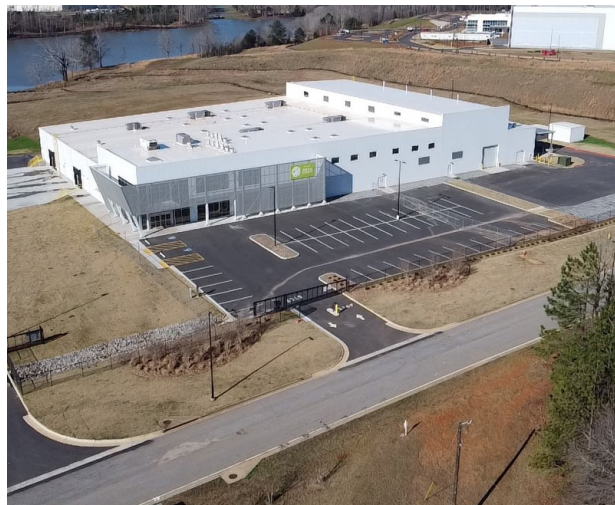
The Lakes at Green Valley, an industrial business park located along the Arthur K. Bolton (State Route 16) corridor.
