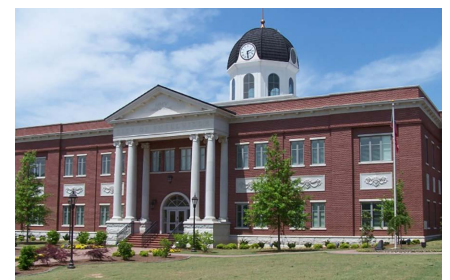
Existing spaces and buildings
