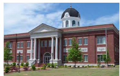
Existing spaces and buildings
