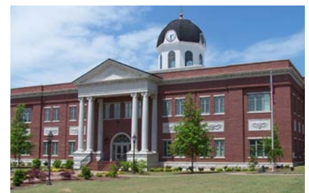
Existing spaces and buildings
