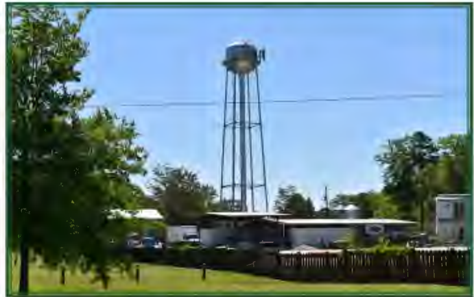
Figure 30. A water tower in Siloam
