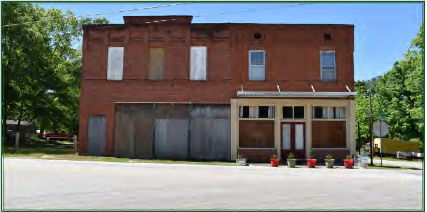
Figure 24. Buildings in Historic Downtown Siloam. The right building was originally the Bank of Siloam
