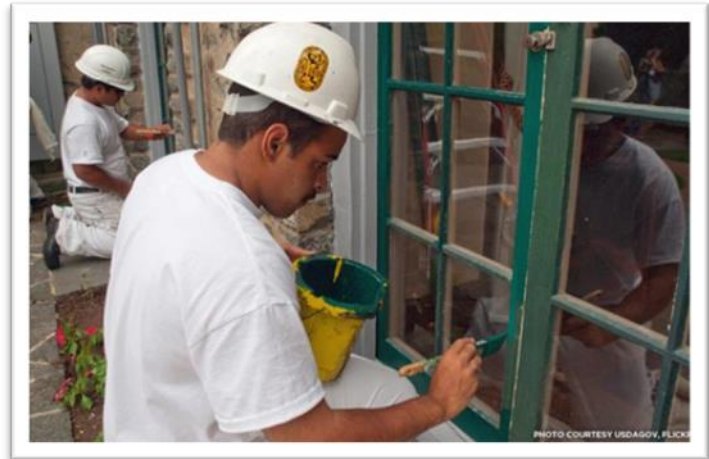
Workers Restoring Historic Windows
