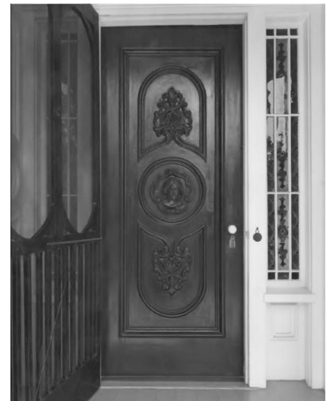
Sam Sawyer House Front Door Detail
