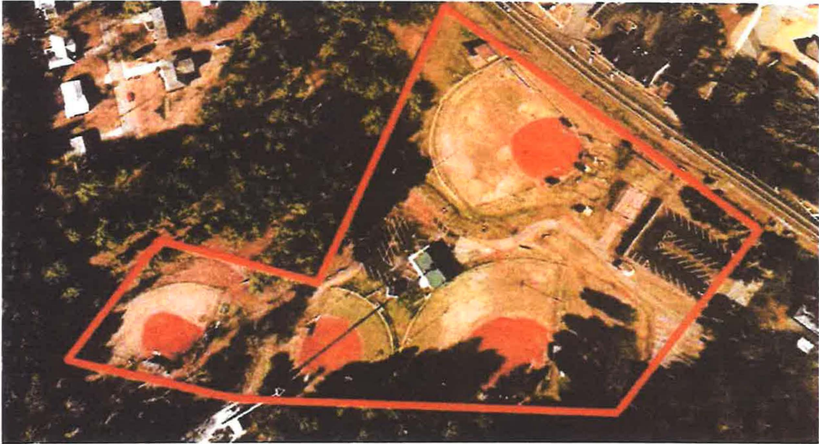
Alexander Park (County is responsible for maintenance of everything inside the Red Lines)
