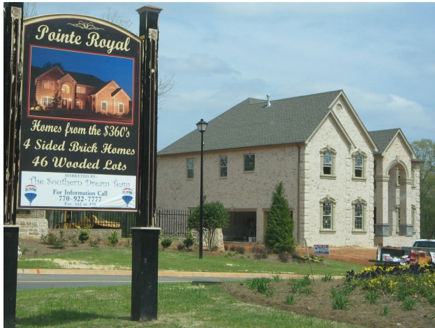
Higher End Housing Under Construction
