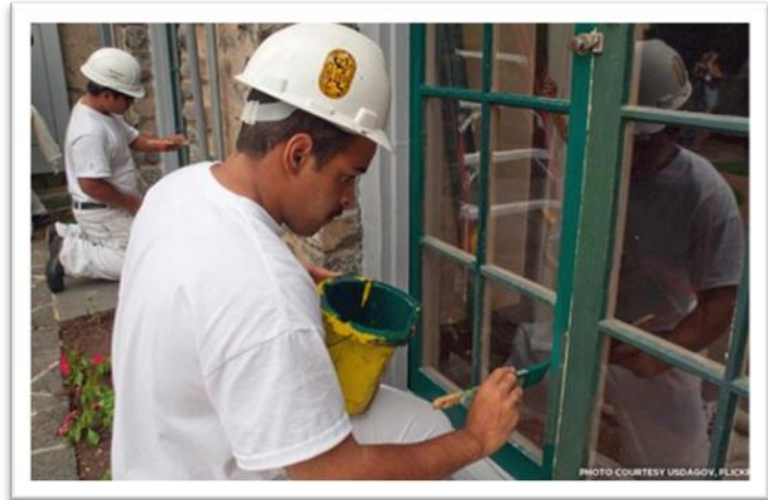
Workers Restoring Historic Windows
