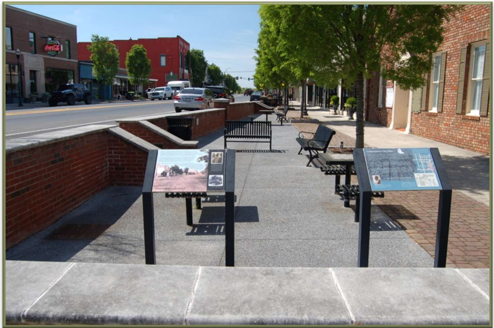
Streetscaping, Main Street, Cedartown
