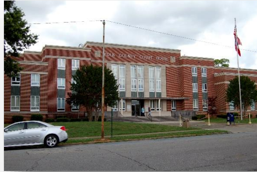
Figure 10. Polk County Courthouse, Cedartown.
