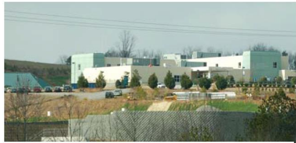
Piedmont Mountainside Hospital
