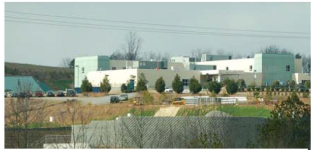
Piedmont Mountainside Hospital
