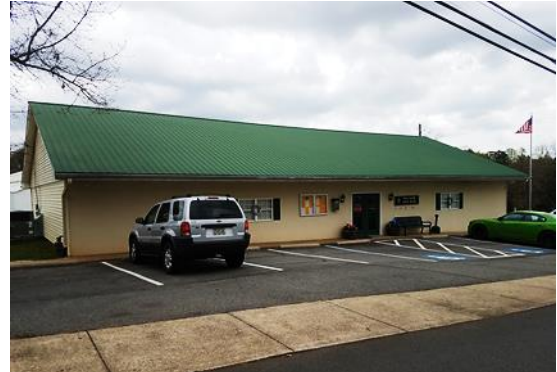
Figure 73: Nelson City Hall along Kennesaw Avenue
