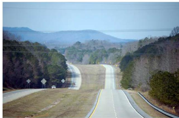
Looking north on Hwy. 515
