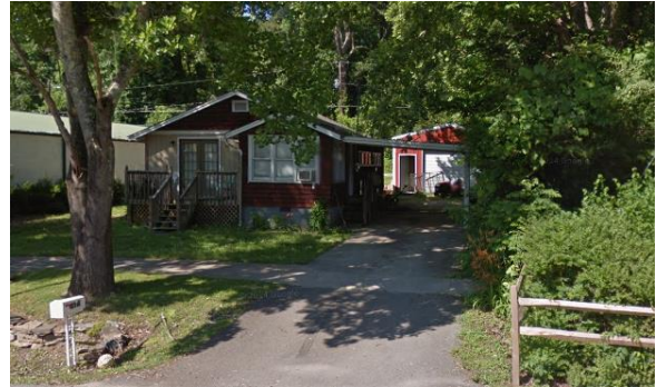
Figure 84: Single family detached residence along Highway 136 in Talking Rock
