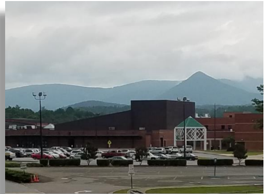
Figure 35: Pickens County High School
