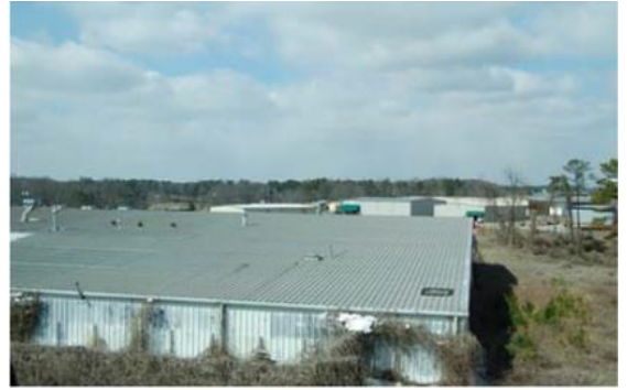
Figure 62: Typical industrial Structure located in Pioneer Industrial Park.
