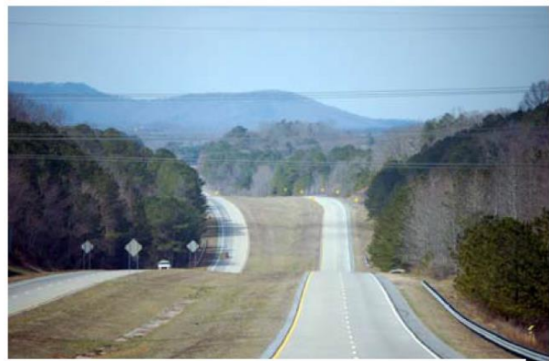
Looking north on Hwy. 515
